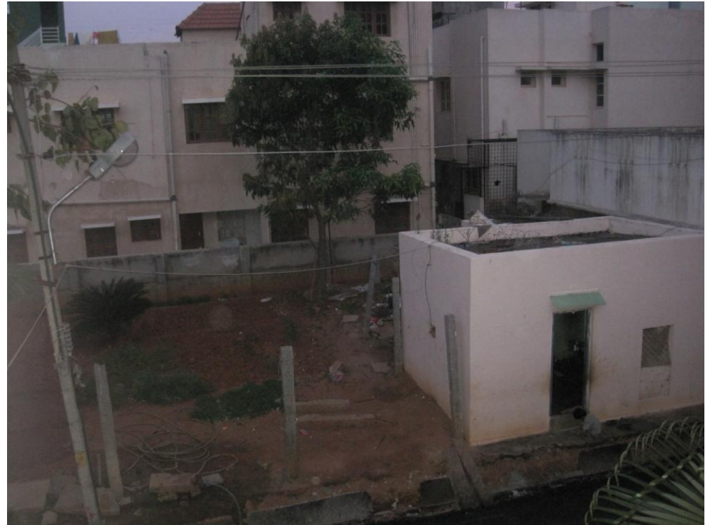
Construction of new school @ PJ
