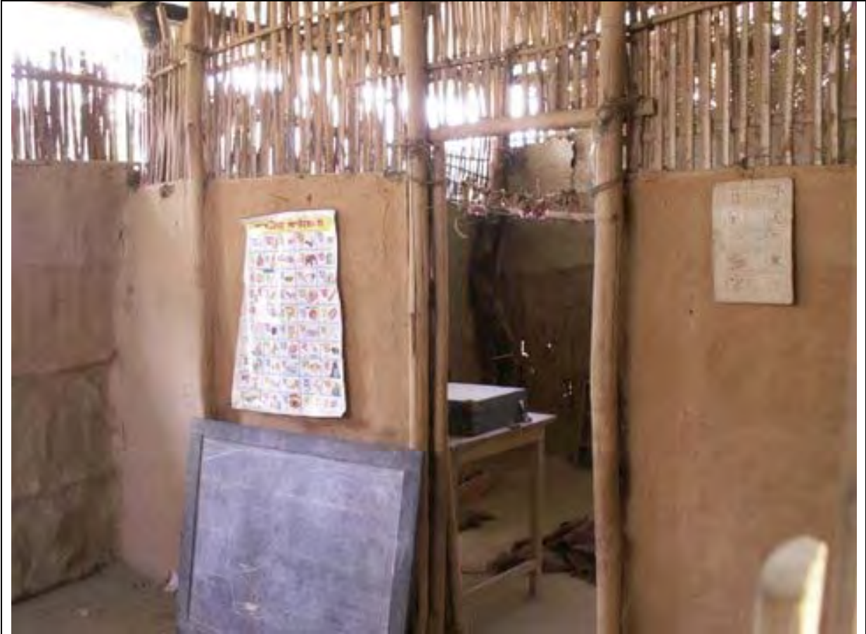
Photo 4: Dikchak Pre-Primary School – View of the inside of the school building
