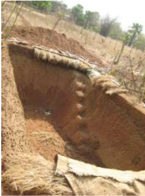
Figure 13: Rain water harvesting structure in the making in Uthnau.
