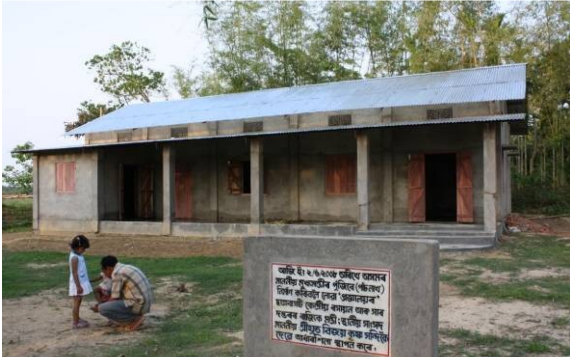
New boys' hostel being built from MLA/MP fund
