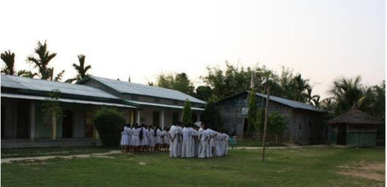
Newly built concrete girls' hostel (the hall with higher roof towards left of center)
